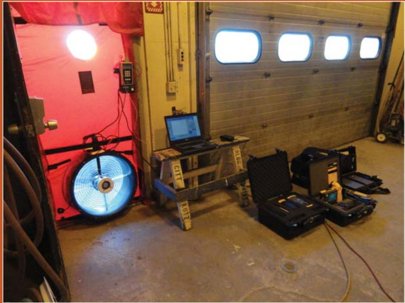
Above, a blower door and building diagnostics at the Public Works building in Kotzebue. Photo courtesy of Renewable Energy Alaska Project.
