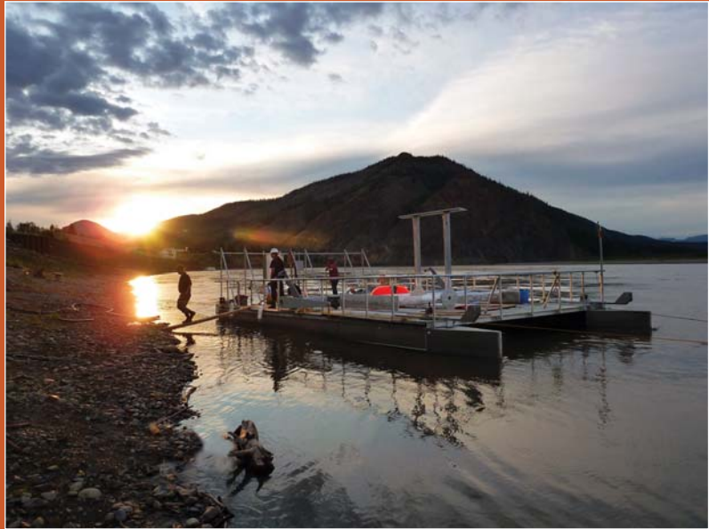
Above, the Yukon River Hydrokinetic Turbine Project. Photo by Mark McCready, Alaska Power and Telephone.
